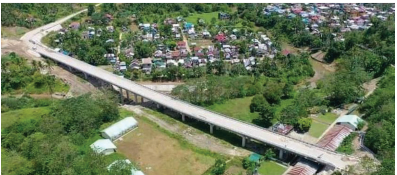
The Php 70 M Jipapad Bridge in Eastern Samar links the Provinces of Eastern Samar and Northern Samar and is expected to curb insurgency in the two provinces. The bridge forms part of the highway that will connect Jipapad to Las Navas, a town in Northern Samar where CTG rebels are frequently sighted, while the town of Jipapad is one of the areas in Eastern Samar also affected by the insurgency
