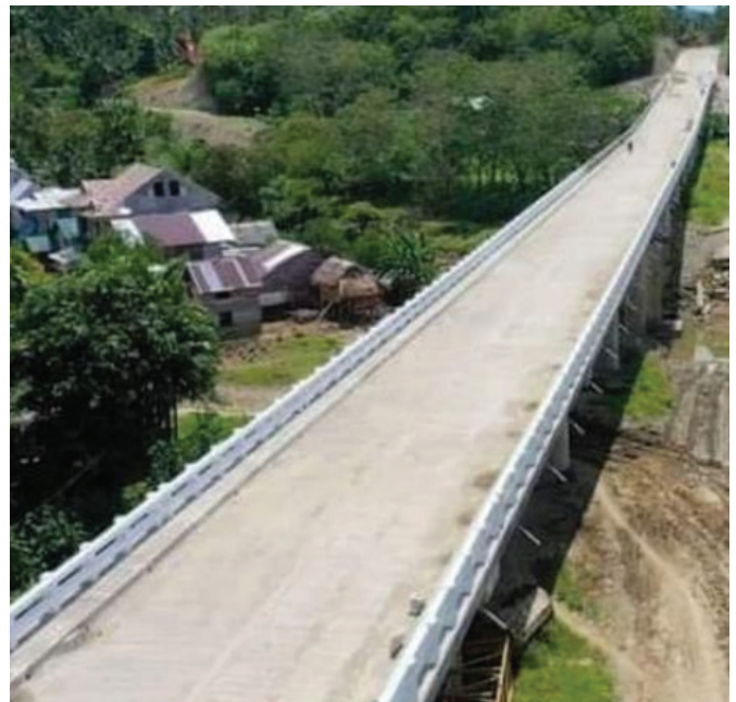
THE PHP 70 M PAMANA-FUNDED JIPAPAD BRIDGE IN EASTERN SAMAR, TURNED OVER ON JUNE 24, 2022, IN EASTERN SAMAR PROVINCE, EASTERN VISAYAS REGION
